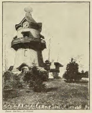
Here is how Greenwich, Connecticut, improved the appearance of an ordinary steel tank. A structure of this kind, if centrally located, could be made to house a volunteer fire department and serve as a town-clock tower as well.
